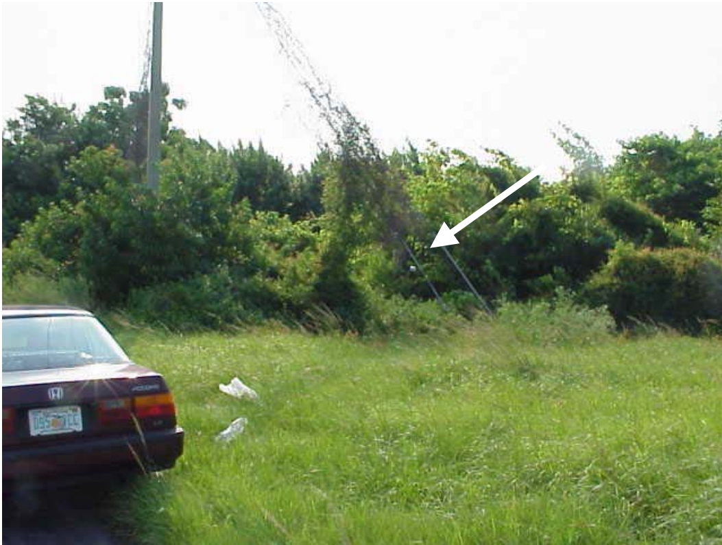
Figure 3. Rain cap and PSD attached to a telephone pole support wire
